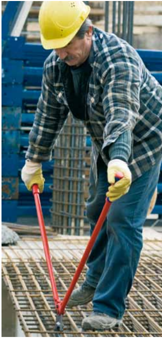
The special shape of the mesh cutter head enables it to cut structural steel that is lying down flat
